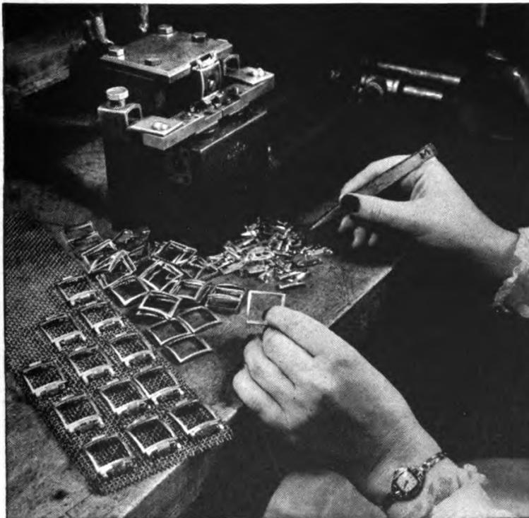
Miniature "spot" welding. The lug is welded onto the bezel of the case by a miniature welding process. These are the skeletons of the watch front.
